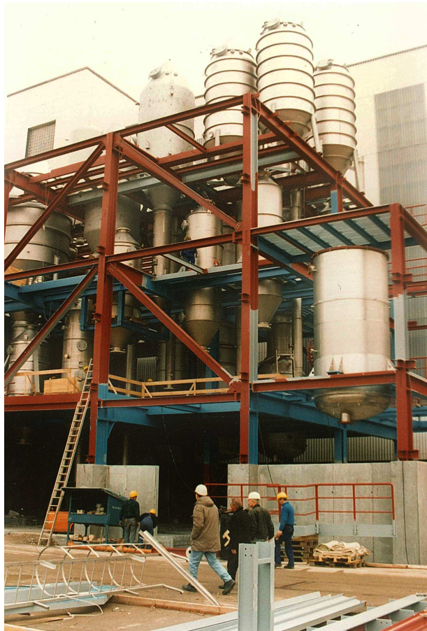
Fig. 5. New 7-effect recrystallization plant at Bad Friedrichshall, under erection
